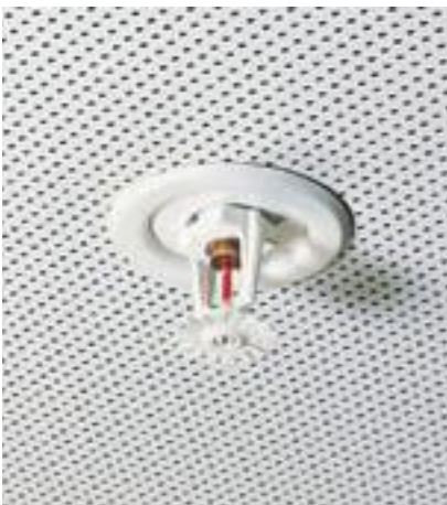
▲ Sprinkler head fitted through circular cut-out
