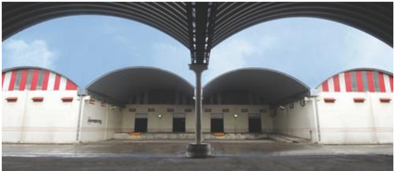
▼ Armstrong Warehouse, Bhiwandi
