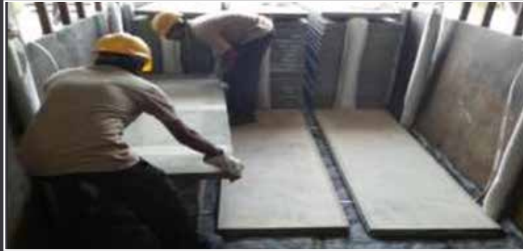
Vpanels under loading in a truck.
