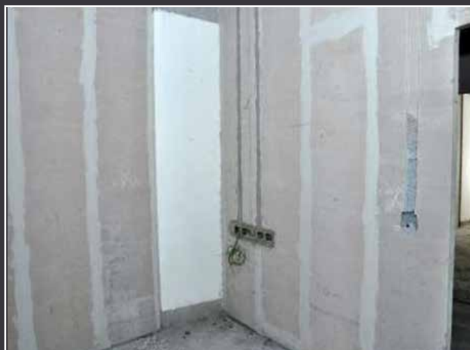
Electrical Conduit work on 75mm thick Vpanels
